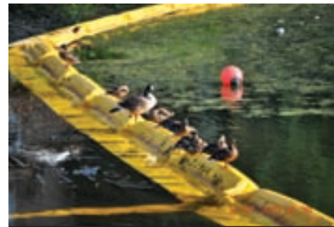
Ducks at Lake Elkhorn have grown used to the site of dredging equipment in and around their habitat. Here, they perch atop a turbidity curtain used to confine stirred-up sediment to the dredging area.
